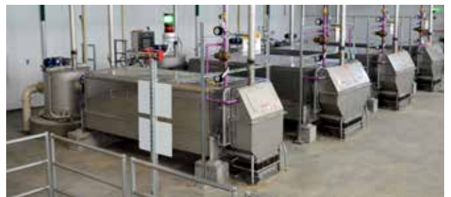
RST Installation West Boise
