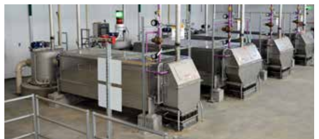
RST Installation West Boise
