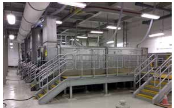
Three BHX-1100 x 6000L screw presses Tacoma, WA
